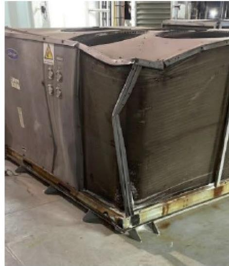
Figure 3: Damage to ACU
