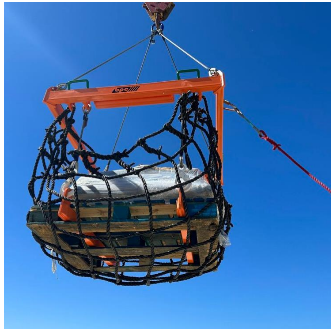
Pallet Lifting with Safety Net
