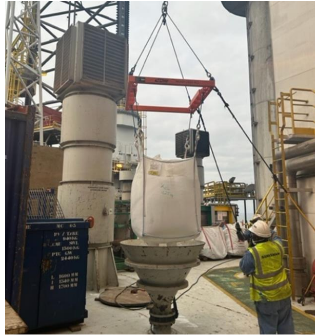
FIBC Lifted with IBC “Spacer” Slings
